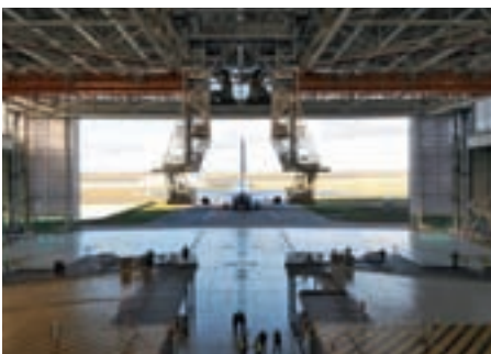
A380 hangar at Roissy-CDG
